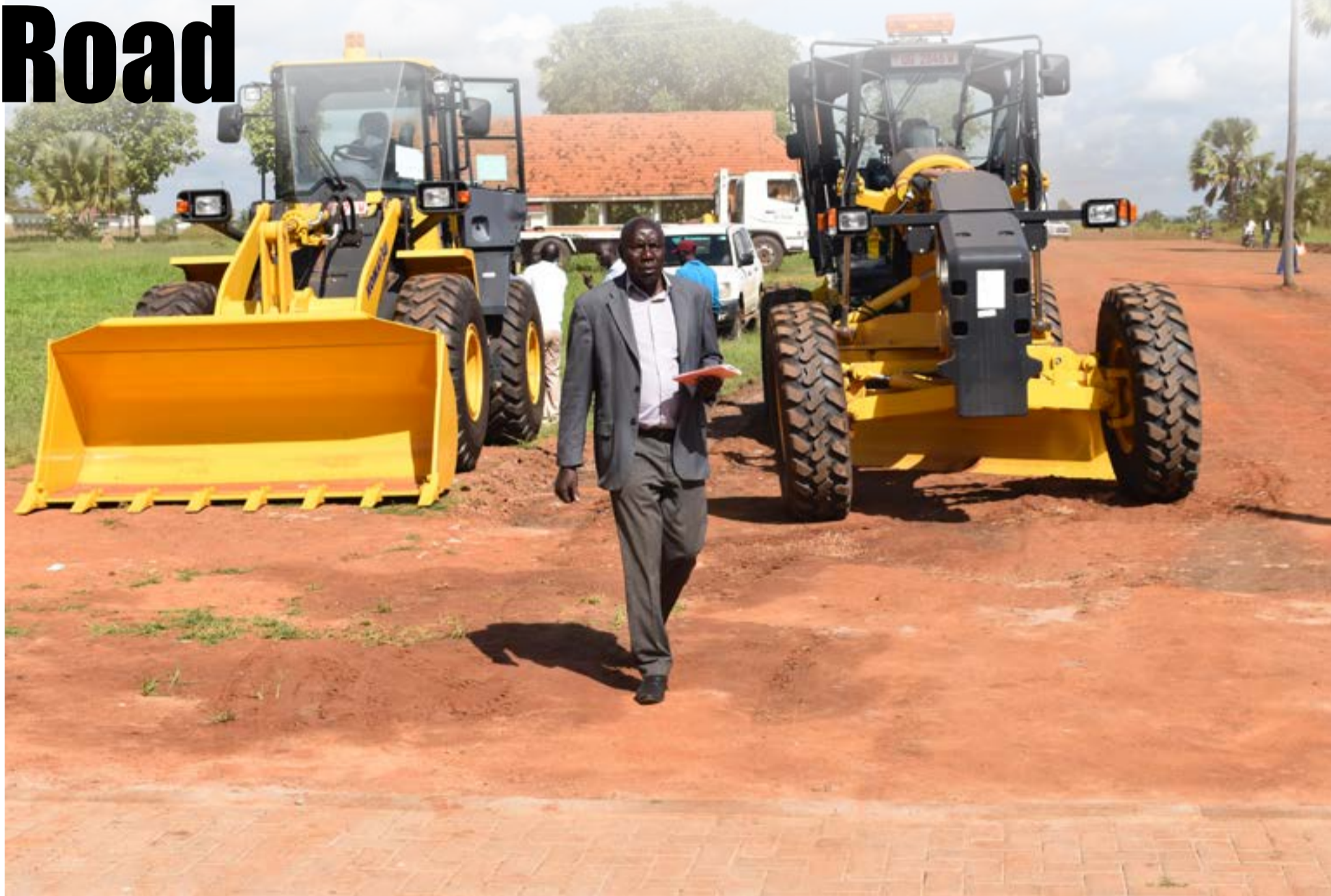
The Secretary for Works in Kalaki District Mr Robin Hood Ekwau inspects the construction of the 500 metre road that connects to district HQTRs from the main road. Photo Julius Odeke
