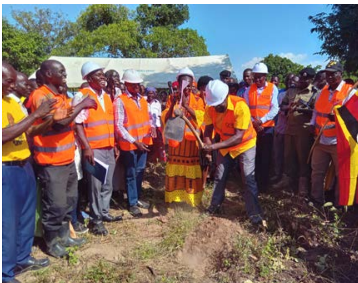
Minister Ecweru breaking the ground for the construction of Amolo Seed SS
